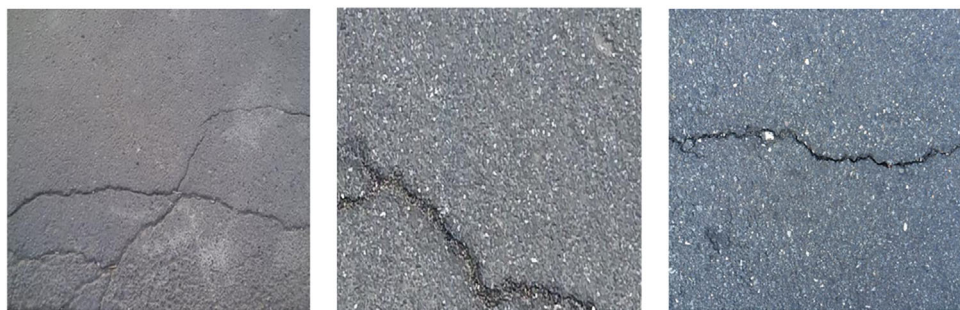
FIGURE 4 Instances of D1. Examples of pavement crack datasets without shadows.
